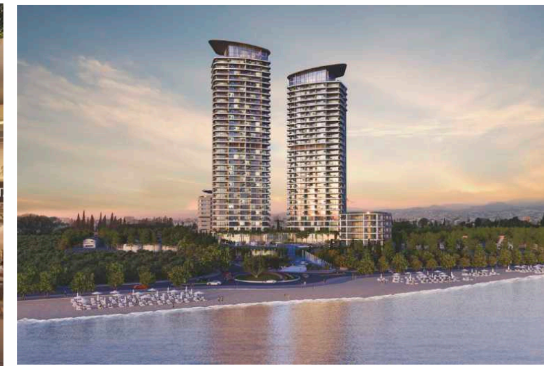
SEAFRONT RESIDENTIAL & SERVICED APARTMENTS
